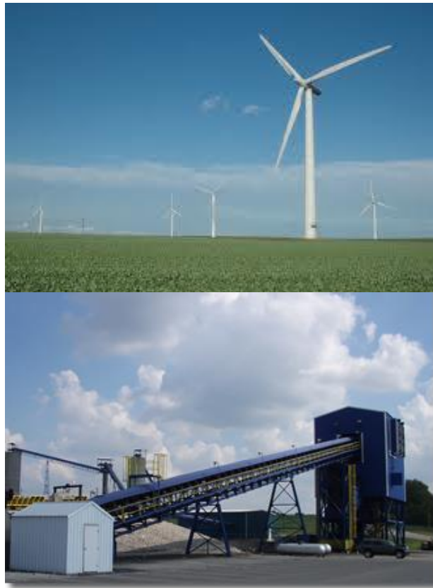
Figure 4 – The Timken Company – Wind Turbine and Coal Conveyor
